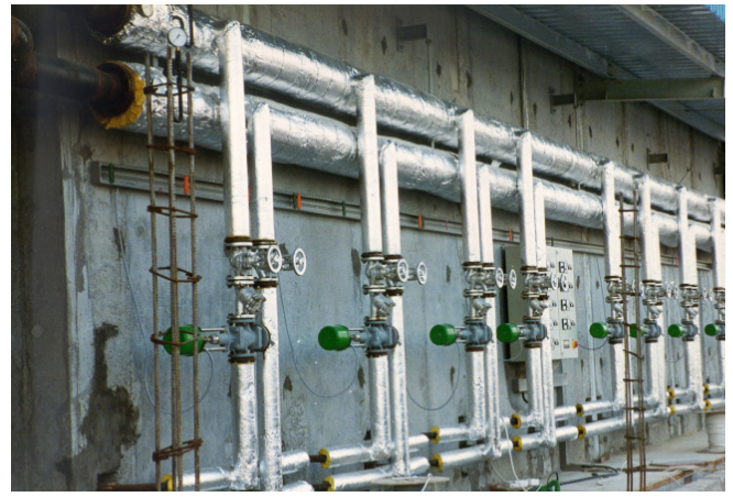
Picture 3: Outside view of a stone curing system with 18 chambers for concrete products with thermal oil
